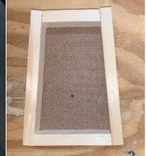
2. Attach  $\frac{1}{2}$ " dowel to top (leave loose) 3. Nail top to frame 4. Glue  $\frac{1}{4}$ " dowel to top
